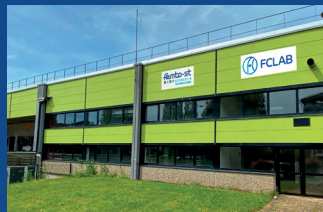
New platform dedicated to electrolyzer testing
